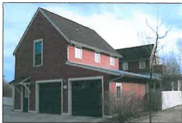
One-and-a-half-story carriage house.
