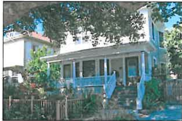
The entry to the right opens to a stair leading to the upper unit, which takes up the entire upper floor. The door to the left opens directly into the lower unit, which takes up the entire lower floor.
