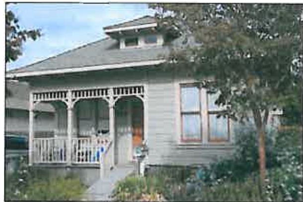
Partial-length integral porch integrated into the overall massing.
