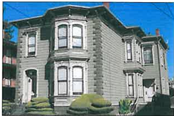
Duplex with both the front and rear unit entries/stoops appropriately engaging and addressing the street.
