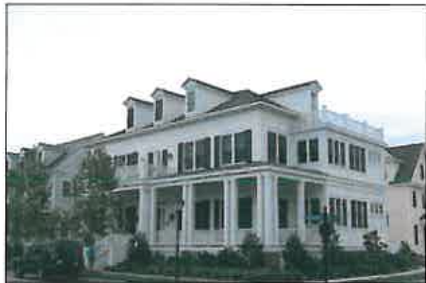
A newly constructed sixplex that is of an appropriate scale and character to be integrated into a primarily single-family neighborhood.
